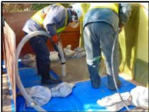
High pressure water cleaning of paved road
