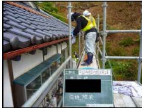
Wiping off a gutter
