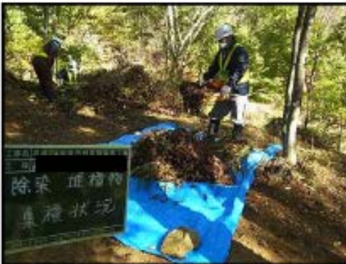
Mowing and removal of sludge
