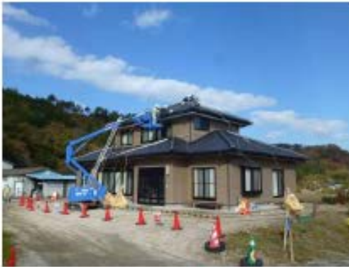
Wiping off rooftop and walls
