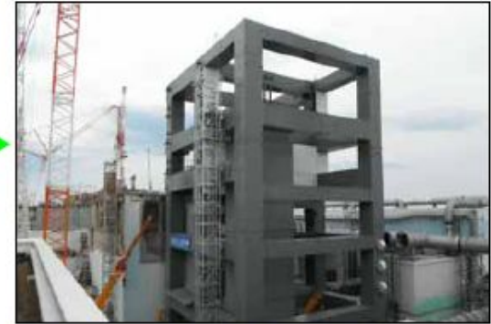
(3) Completion of the steel frame construction excluding the upper part of the Reactor Building (April 10, 2013)
