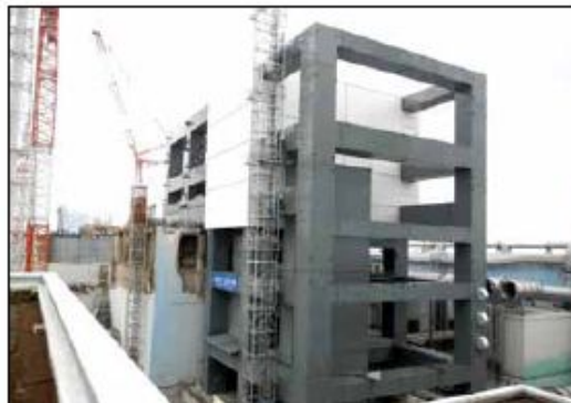
(4) Completion of the steel frame construction (May 29, 2013)
