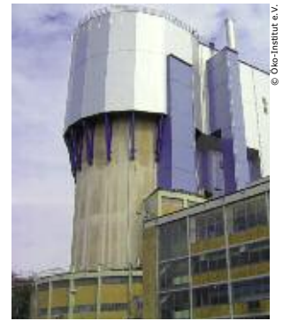
The AVR pilot reactor with the "material sluice" attached to the reactor building, where the reactor vessel is to be lifted out, tipped and loaded onto a freight vehicle.
