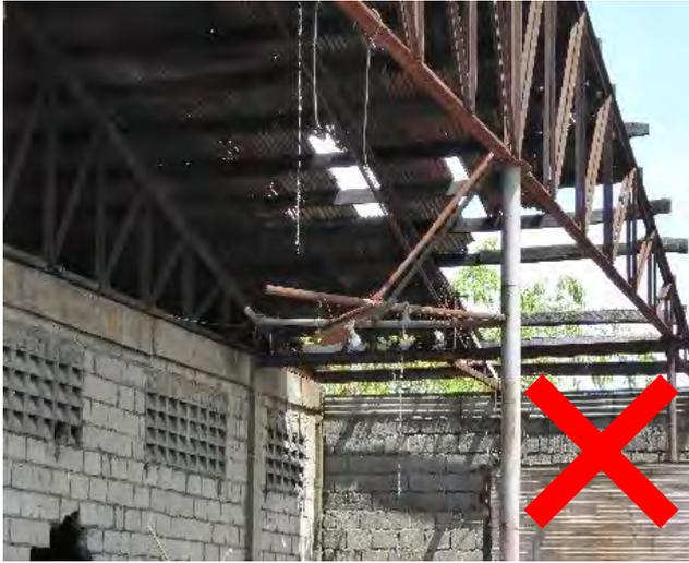
A steel corrugated roof above a smelting operation corroded from sulfurous compounds.
