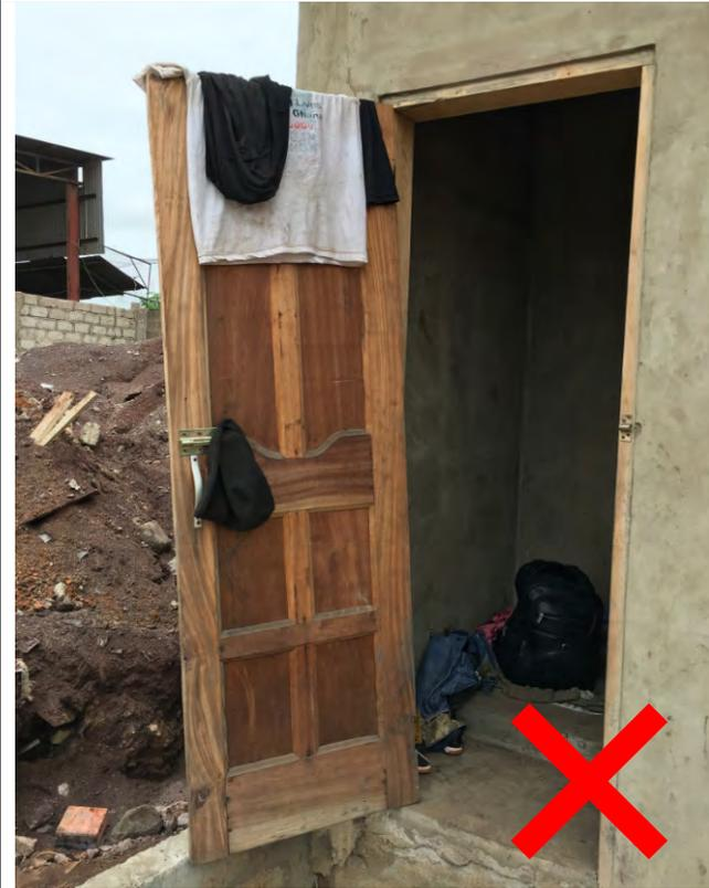
This changing room is provided for workers but is not equipped with any lockers or a shower and in the absence of any one-way system there is every prospect that contaminated working clothes will come into contact with clean clothes.
