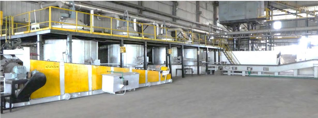
*Elevated lead refining kettles with a gravity feed to casting machines adjacent to kettles 1 and 4*
