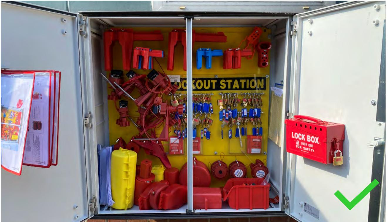
Lock off / tag out box. This box contains all the keys, locks and tags for effective isolation control. There is also a manual to inform engineers of the appropriate type of lock required for each item of plant and where to apply the isolation.
