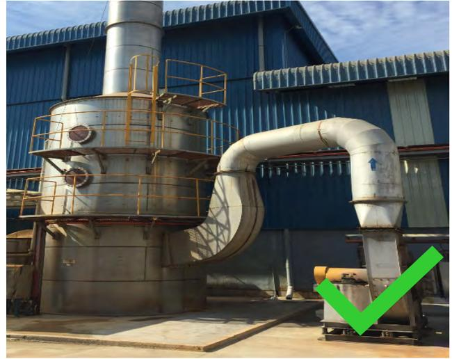
A scrubbing tower removes residual sulfur dioxide from the off-gas stream (sulfur removal method 3).
