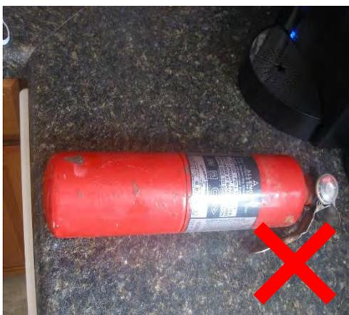
This fire extinguisher has been left on the floor where it might be damaged or triggered if someone trips over it. The fire extinguisher should be wall mounted and if that is not possible, inside a floor stand.
