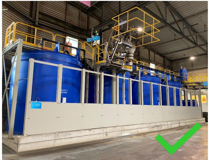
An Effluent Treatment Plant (ETP) will capture any process effluent, including any battery electrolyte arising from battery breaking and either neutralises the effluent for a controlled and legal release or converts the effluent into a saleable product or non-hazardous waste. Any residual liquid is used to either cool the lead ingots during casting or for damping down dusty work areas.
