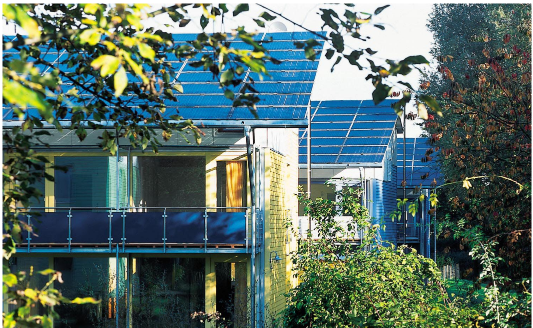
PlusEnergy houses in Freiburg (Source: Rolf Disch architects)
