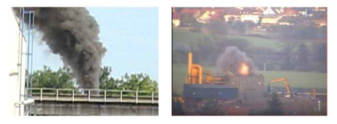
Figure 10 Emission from a shredding plant during a deflagration (BREF WT, 2017)
